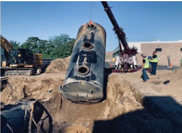
Photo: UST Removal at Main Street Site
