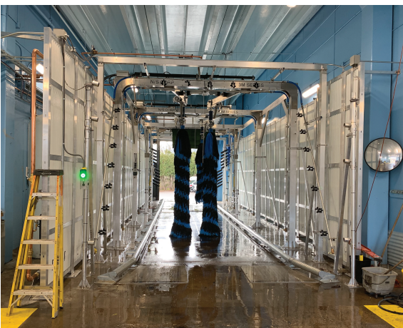
Photo: New Bus Wash Installation at Northampton Garage
